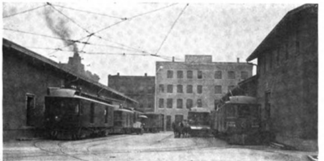
TYPICAL SCENE, INTERURBAN FREIGHT STATION, INDIANAPOLIS
